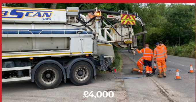
Great Alne flood alleviation project
