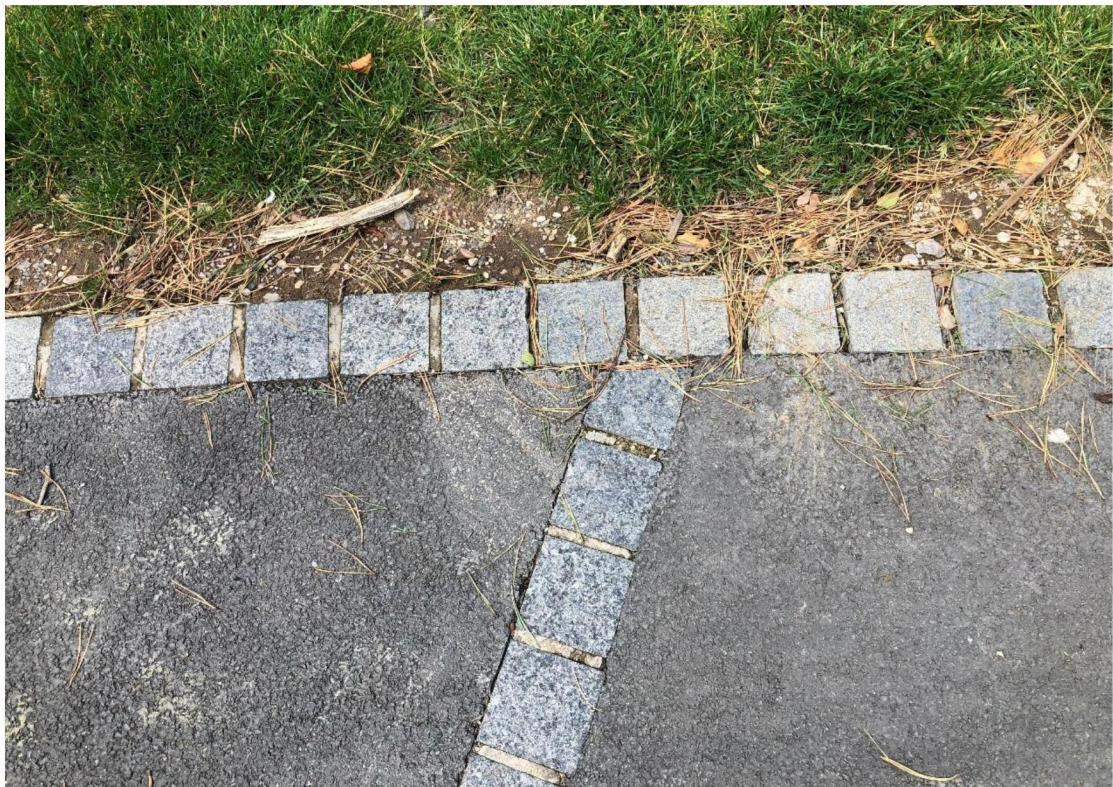
P4 – Detail of Granite Setts Edging
