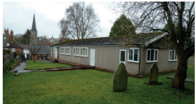
Baptist Hall, behind Baptist Church, High St.
