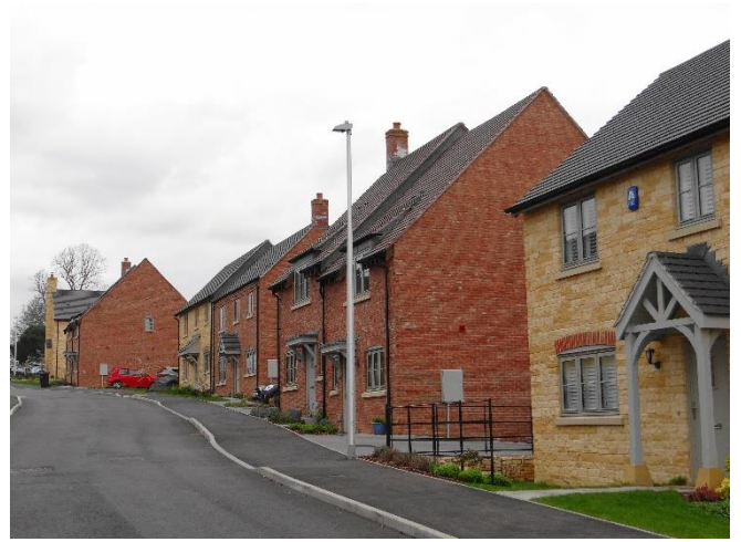
General view looking west
