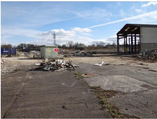
Site clearance prior to re-development
