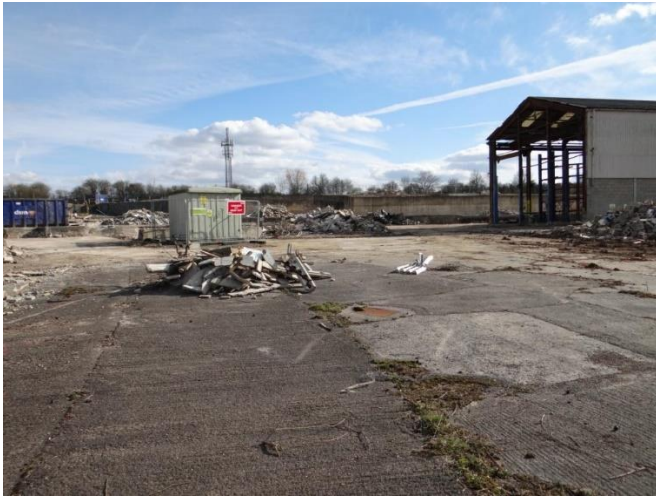
Site clearance prior to re-development
