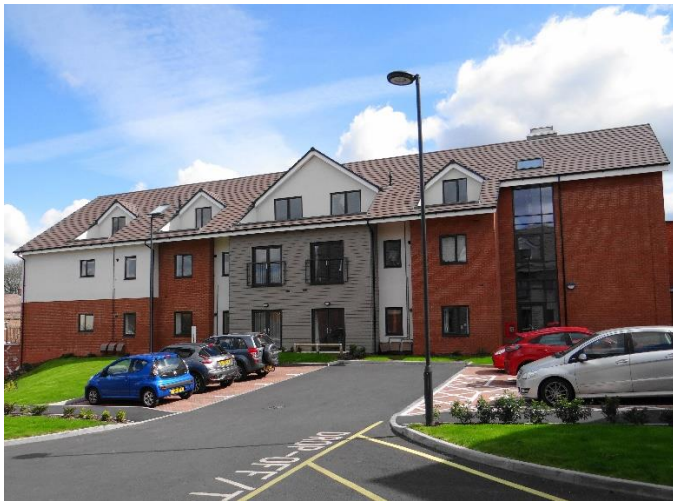
View looking east
