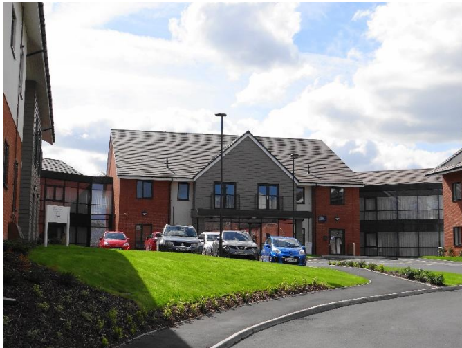
View towards main entrance
