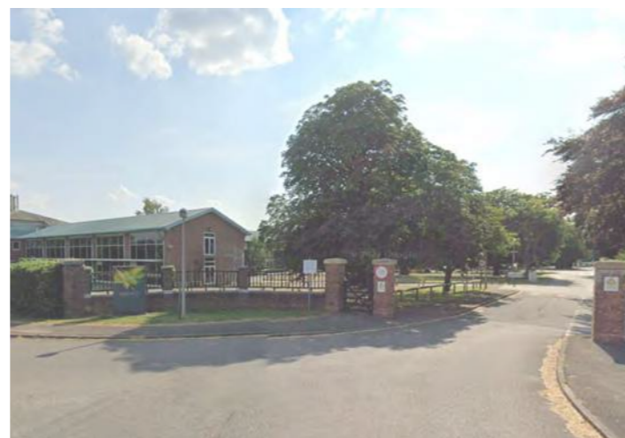
5 A429 MAIN ENTRANCE TO SITE
