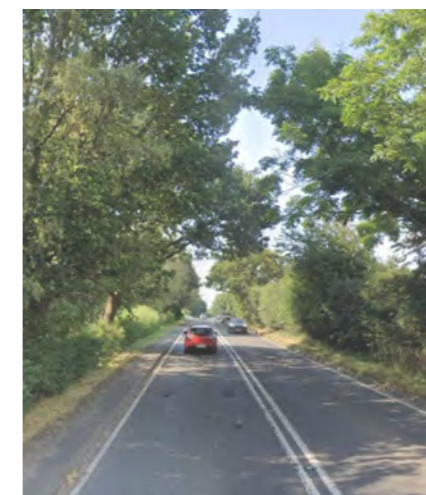
6 A429 SOUTH APPROACH TO SITE
