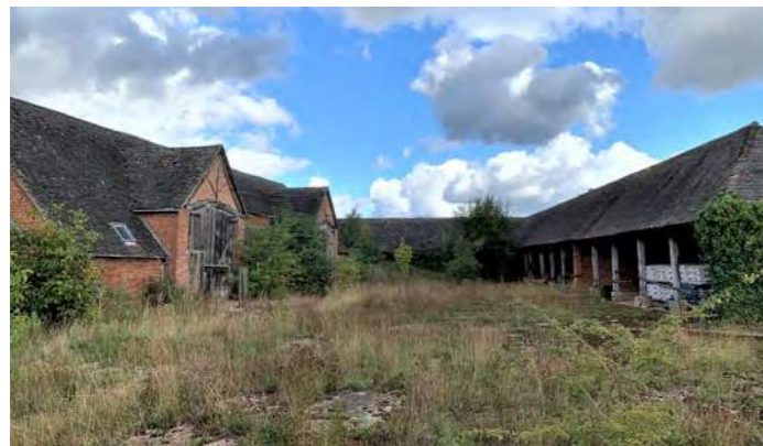
EXISTING BARN RANGE
