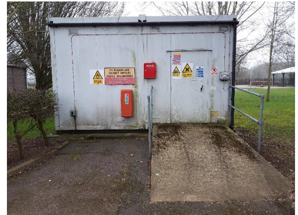
Figure 2.6: Chemical waste store in the west of the campus.
