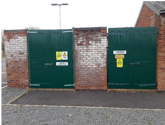
Figure 2.5: Substation, one of at least three, centre of campus.
