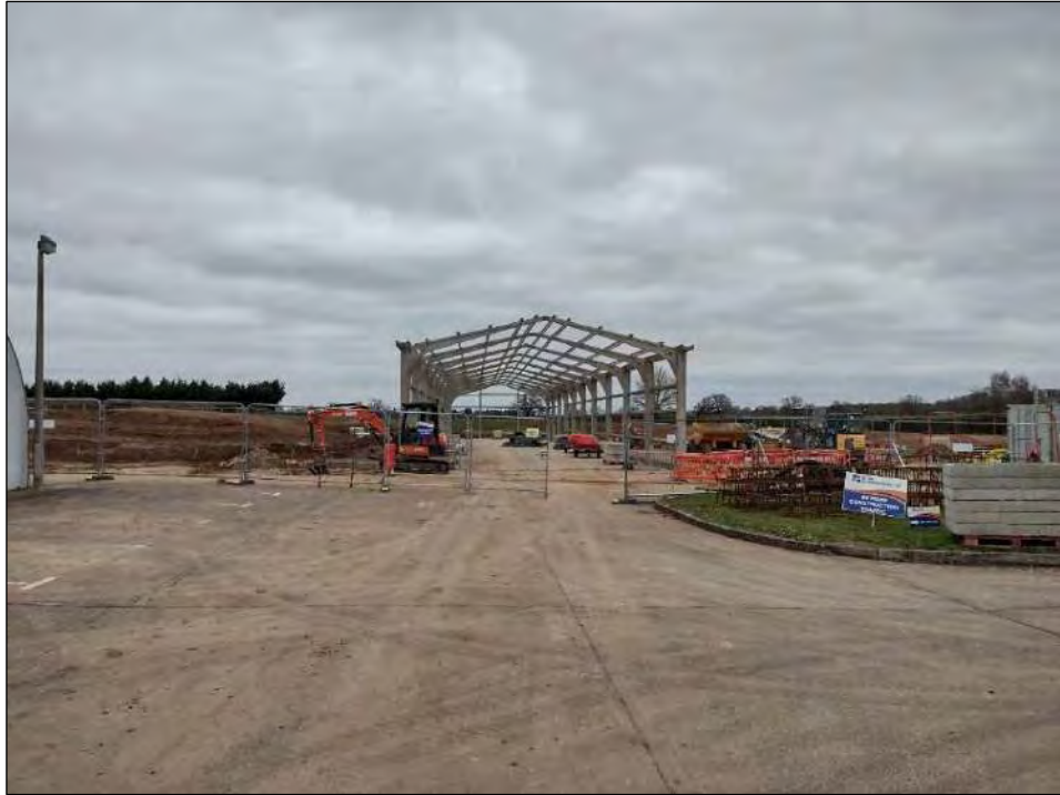
Photo 1 The campus facing north
