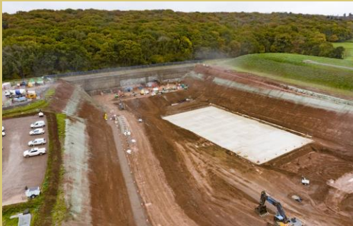
Figure 52: Image of HS2's extensive Long Itchington Wood Tunnel construction site.
