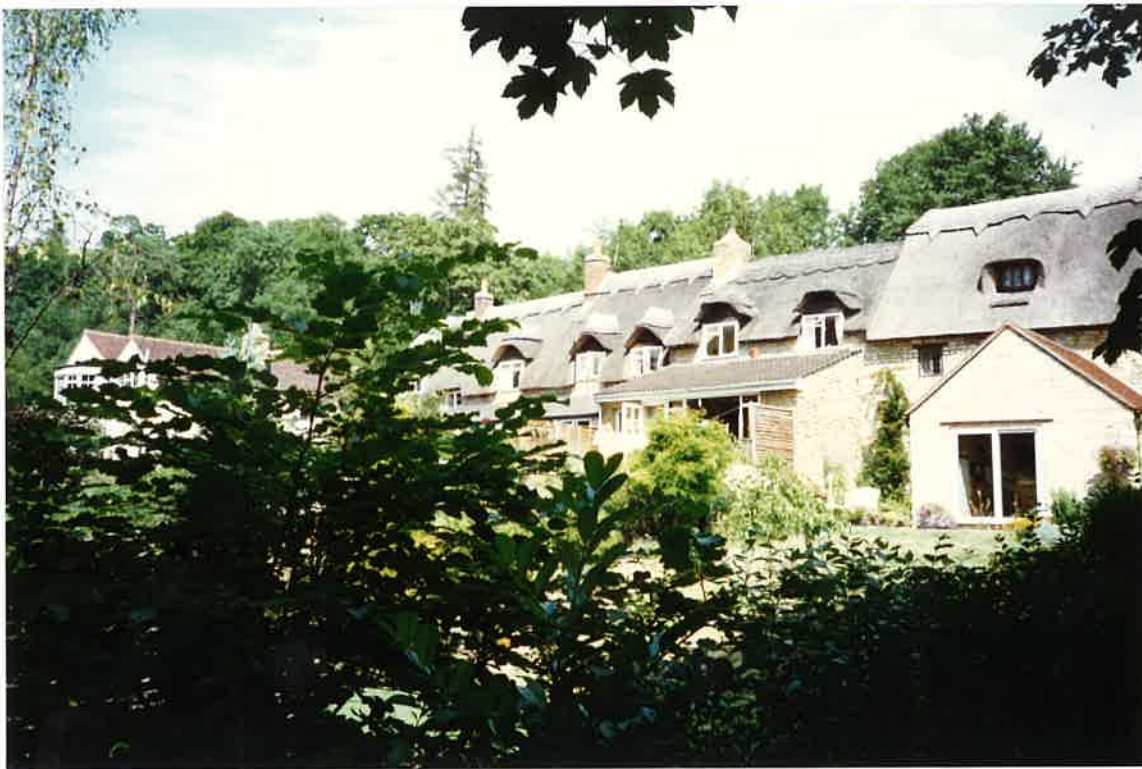
^^ Rear of buildings ref - 116/117
