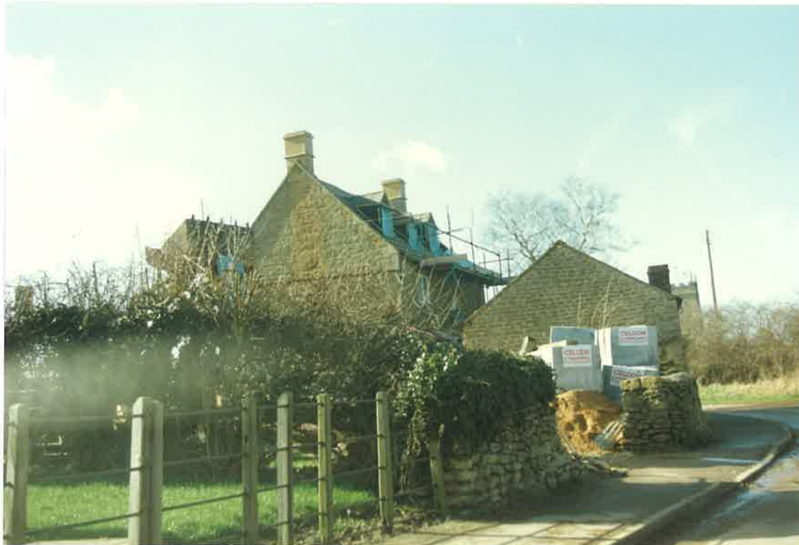
(Key building on corner - undergoing extensive renovation)
