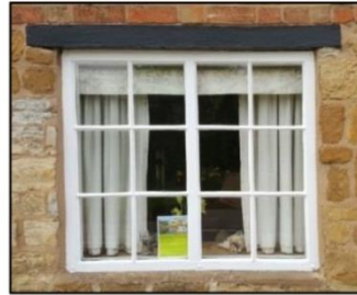
Stone & timberlintels (some stone tile sill)
