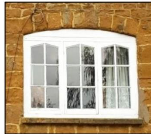
Brick & stone arches above windows – some stone sill
