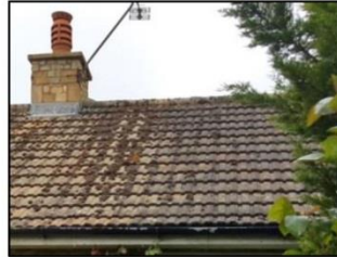
Ironstone clad chimney but with uncharacteristic interlocking clay tile roof
