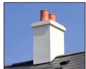
Rendered or painted breeze block chimneys
