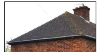
Shallow roof with hipped structure
