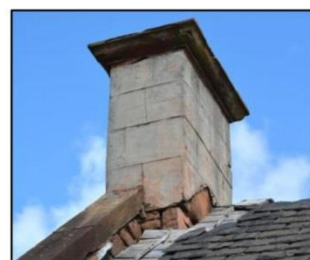
Rendered or painted breeze block chimneys
