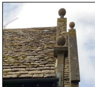
Manor stone verge capping on parapets
