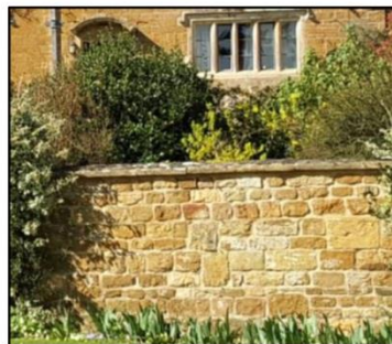
Low ironstone wall - flat top
