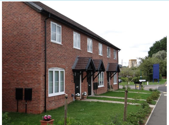
Terrace of 3 x 3 bed houses, fronting Armscote Road
