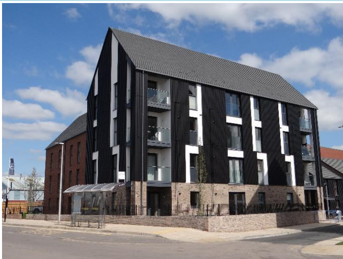
Block of 18 x 1 bed flats for affordable rent
