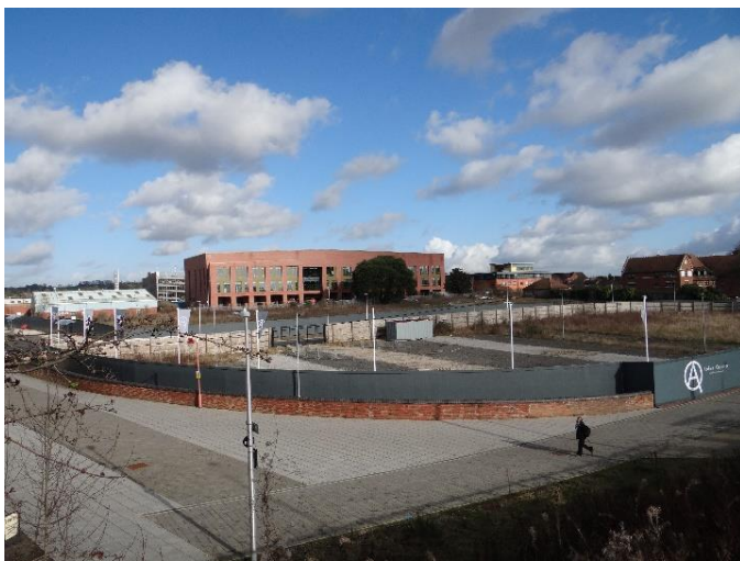
Site prior to redevelopment
