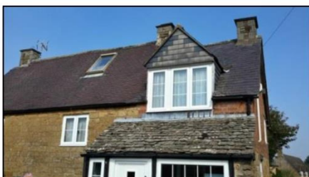
High pitch with chimney at the end(s)
