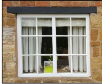
Stone & timberlintels (some with stone tile sill)
