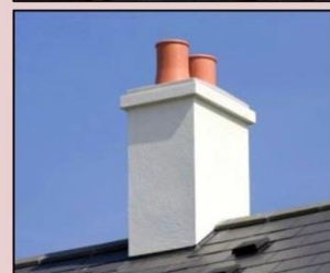
Rendered or painted breeze block chimneys
