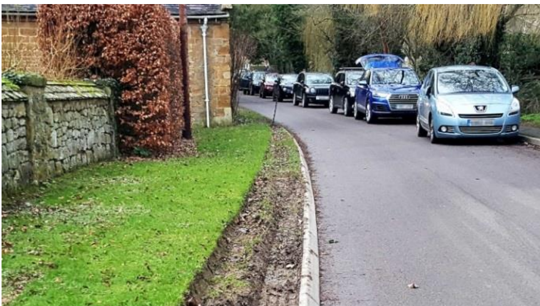
Traffic congestion, parking and associated verge damage on Back Street
