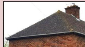
Shallow roof with hipped structure
