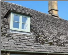
Stone roof and chimney
