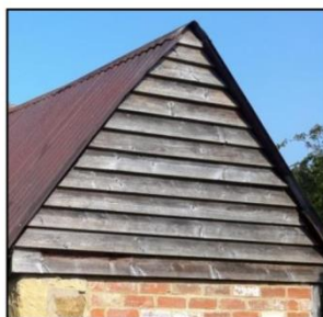
Timber Weatherboard
