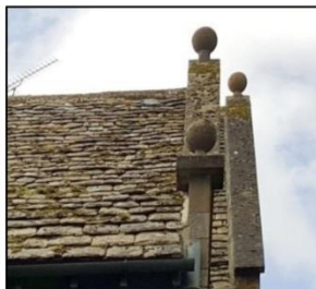
Manor stone verge capping on parapets
