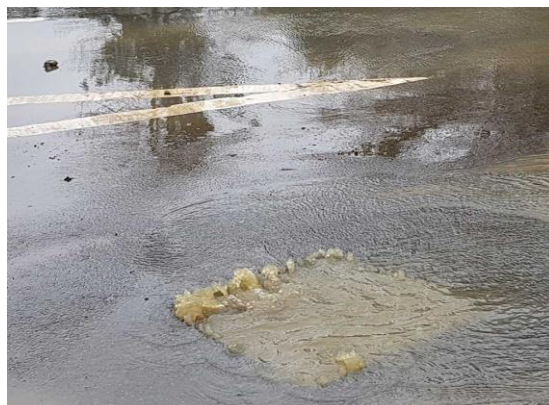
Images of flooding on the corner of Armscote Road and Front Street Including image of flood water coming up through a manhole cover
