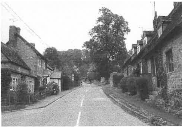
Frontage onto village street
