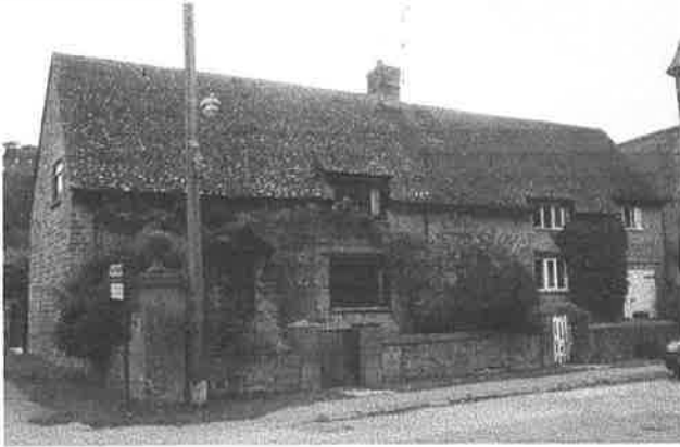
St. Annes Cottage, Church Cottage
