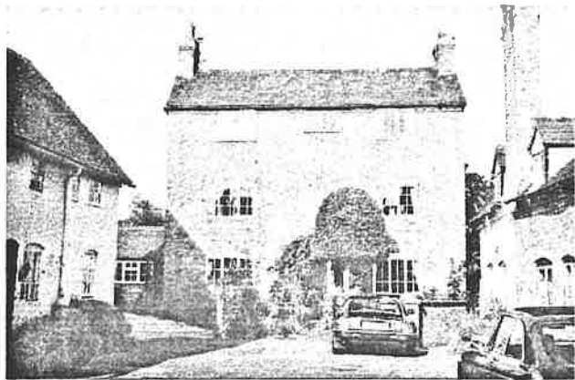
No. 28 Village Street
