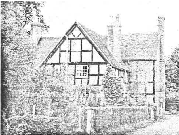
Timber framing to the old post office
