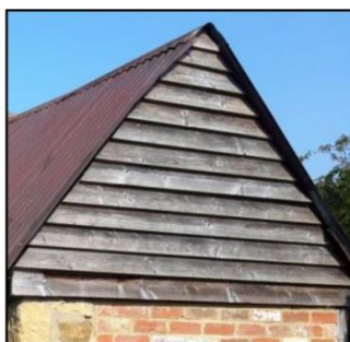
Timber Weatherboard
