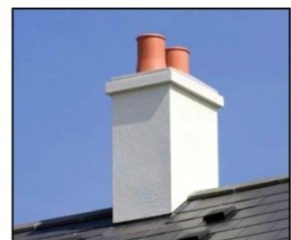
Rendered or painted breeze block chimneys
