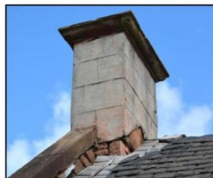
Rendered or painted breeze block chimneys
