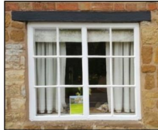
Stone & timberlintels (some stone tile sill)
