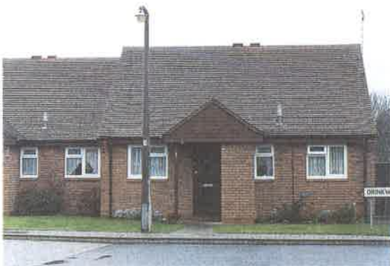
Pensioners' bungalows at Drinkwater Close
