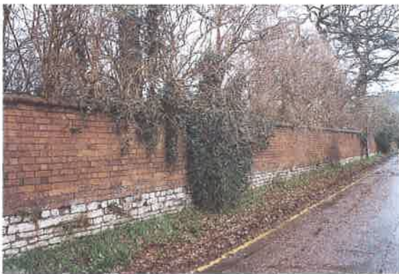
Old red brick wall on stone plinth with terracotta coping
