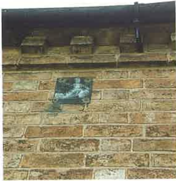
Fire Plate, Spiked Brackets, Dentil course to eaves. 35 Farm Street.
