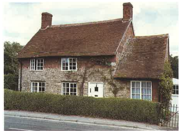
Merevale House, South Parade; coursed stone walls with brick gable, tiled roof, extension to side and boundary hedge.
