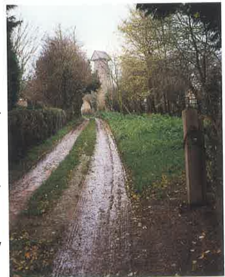
Mill Lane looking south to the Windmill
