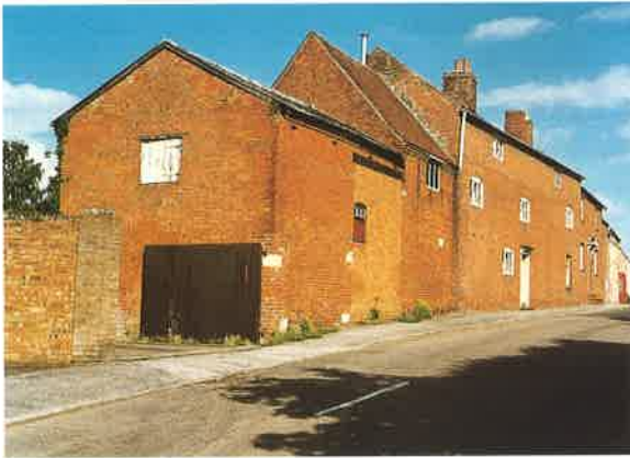
Chesterton Farm, Mill Street.
