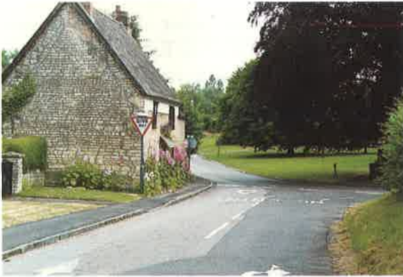
Orchard House, opposite the Pound with raised roof-line in brick and stone. Note the courses of painted brick below the eaves and the splendid Copper Beech on Pound Green.
