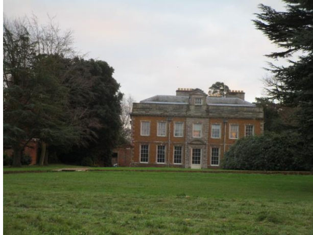
Side of Farnborough Hall from Sourpool Pond (Lakes)
