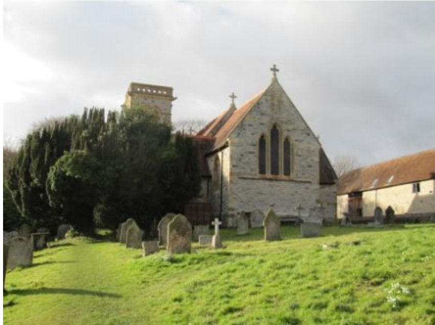
St Peter's Church – rear view
