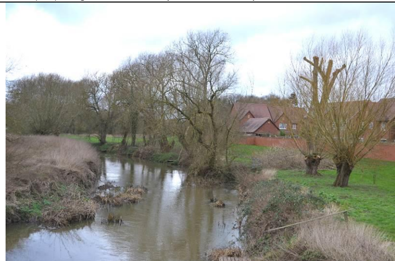
Photo 5. View from bridge on road to Dunnington looking north up the River Arrow and tree cover on the Parish boundary and to flood defences and new houses in Miller's Bank, Broom
