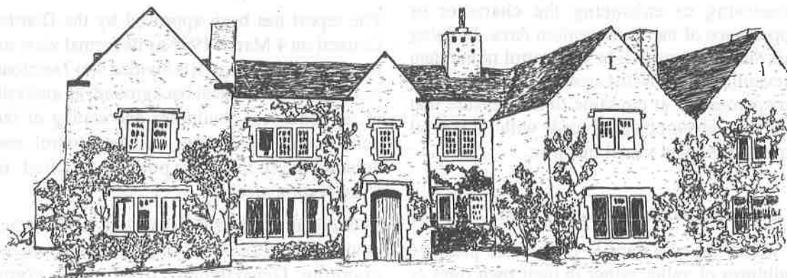
Moat House Farmhouse
