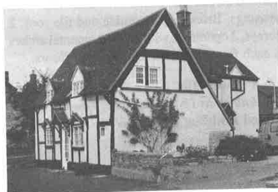
5 Icknield Street (Listed Building Ref No. 10/55 - Grade II) (Now named Old Ford Cottage).
