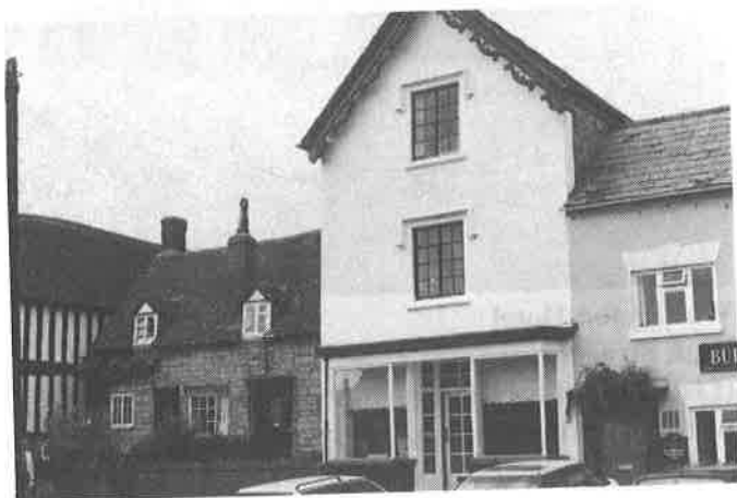
38, 40 & 42 High Street The Old Cottage (42) [Formerly listed as Ryecroft and No. 42 High Street] (photo also pages 7, 10, 15 and 37) (Listed Building Ref No. 10/39 - Grade II) List description : Row of 3 cottages and shop; Nos. 38 & 40 occupied as single dwelling and
