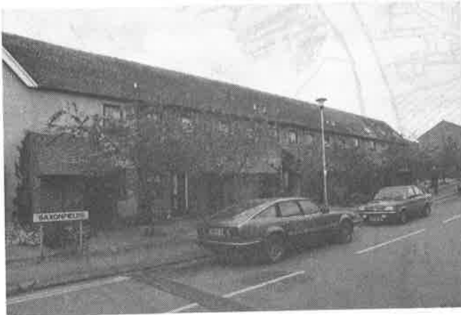
1, 3, 5, 7, 9, 11 & Barn House Saxonfields (photo also page 18) (Ref No. 95) Terraced dwellings, two storeys, plain tile roof, brick, appears to be conversion of former farm buildings.
