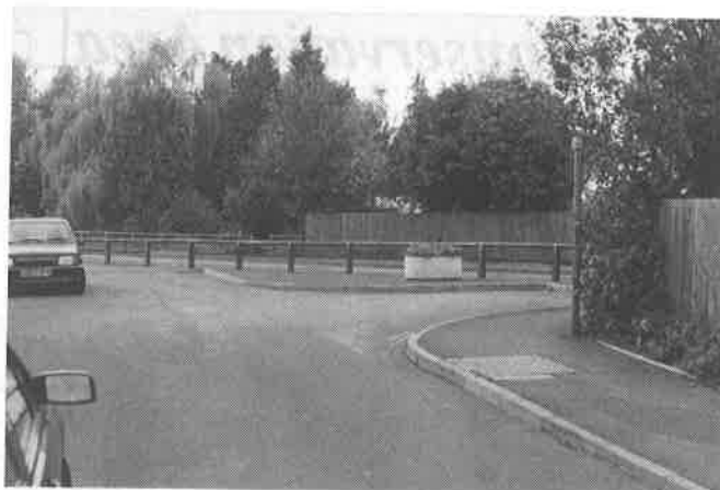
Turning head at the western end of High Street
