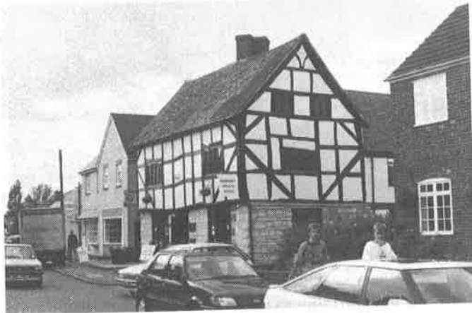
90 & 92 High Street, sympathetically restored
