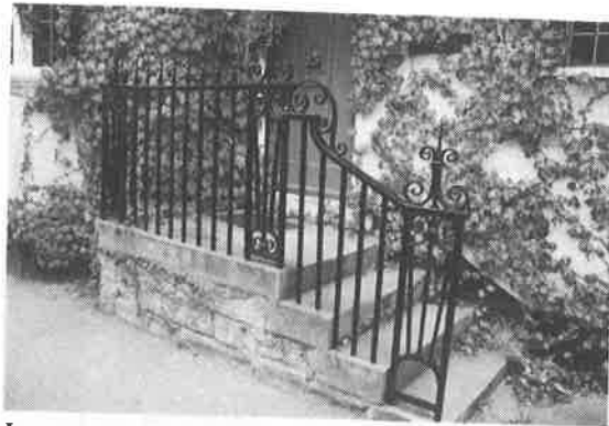
Iron ornamental railings/boot-scraper contributing to the character of High Street
