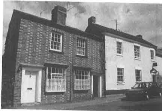
6 & 8 High Street (photo above, left) (Listed Building Ref No. 10/35 - Grade II)
