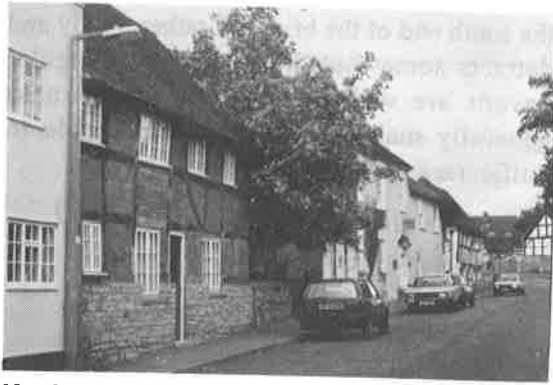
North side of High Street
