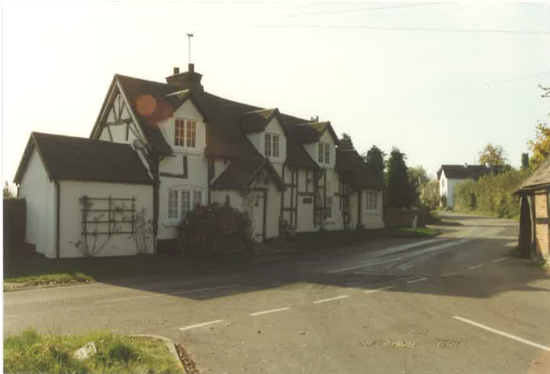
(Rather heavy dormer window additions)
