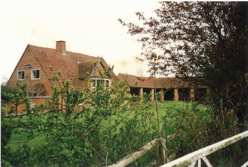
Open Shelter Shed, Jackson's Farm Off Main Street Map Ref - 108, [ 62t ] Farm building, probably C19, one storey, 'L' plan, hipped plain tile roof, brick with brick columns
