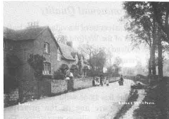
View south east of Field Dyke House and The Grove - circa 1900 (SBT)
