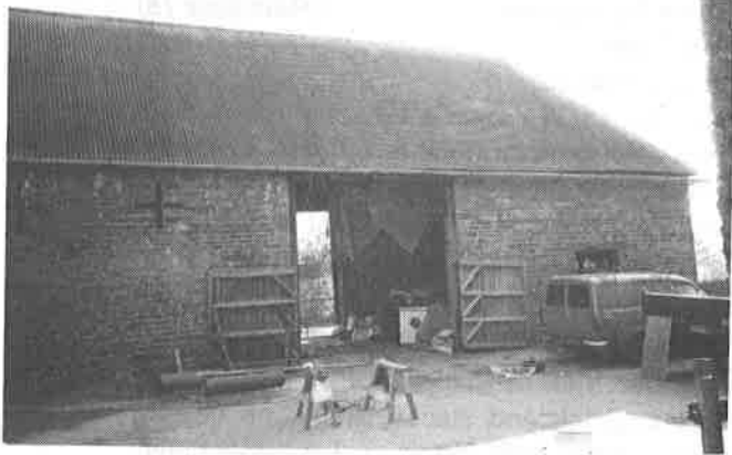
Barn approx. 25m south of Plumtree Farmhouse
