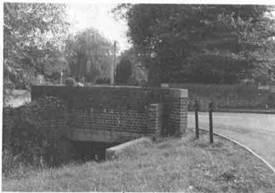
Bridge over Sutton Brook, access to Orchard Close unsuitably planted in the small front gardens of the houses. The access road is carried over a new red brick bridge, the crude design of which contrasts unfavourably with the adjacent stone bridge carrying the main road.
