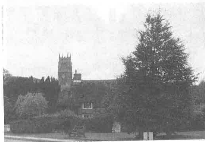
Glen Cottage fronted by a former part of the green
