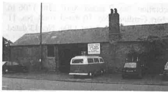
centre to left has plank half doors and wood frame. Plank loft door to left.
