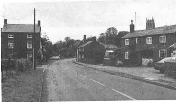
Lytham House and Lavender Cottage, High Street
