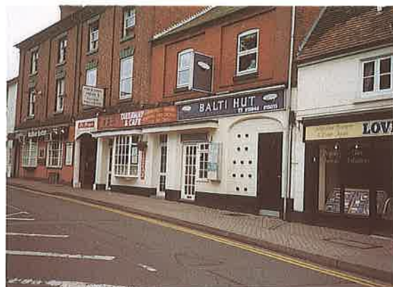
Shops in High Street
