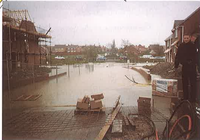
The Southam floods April 1998
