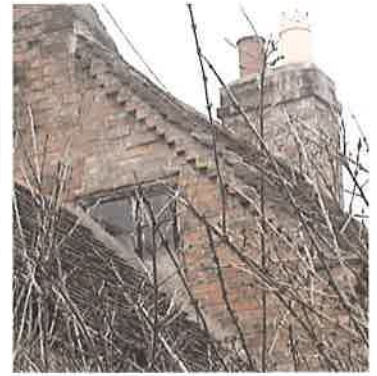
Roof detail, Ashorne
