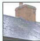
Slate with brick chimney
