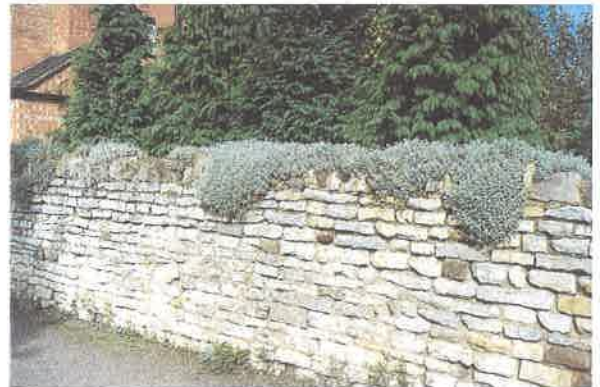
Harbury stone, coursed rubble wall with stone coping.
