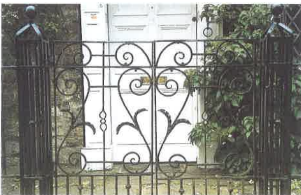
Splendid wrought iron gateway to Wisset Lodge, Church St.
