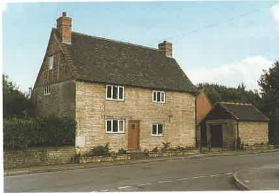
Timber framed gable end, brick chimneys, stone and brick, small windows, converted outbuilding - 27 Farm St.
