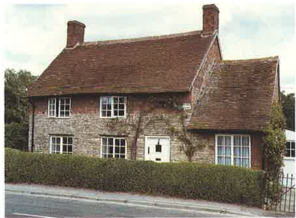
Merevale House, South Parade; coursed stone walls with brick gable, tiled roof, extension to side and boundary hedge.
