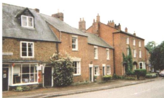
Varied roof lines and periods in the middle of the Conservation Area
