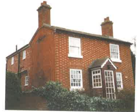
Jasmine Cottage showing decorative brick work
