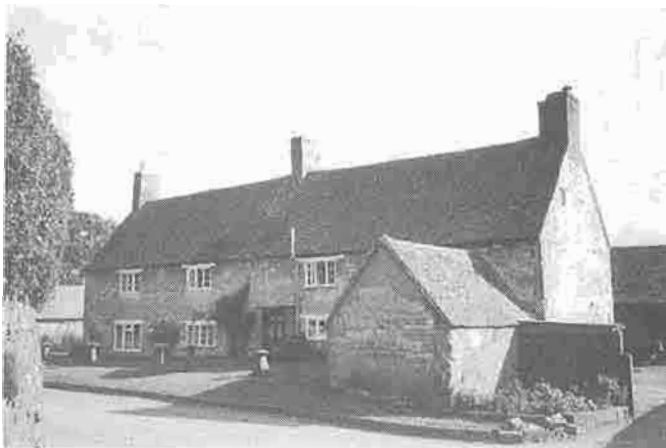
Stone House Farmhouse
