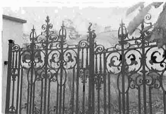
Fine wrought iron gates with poor pillars
