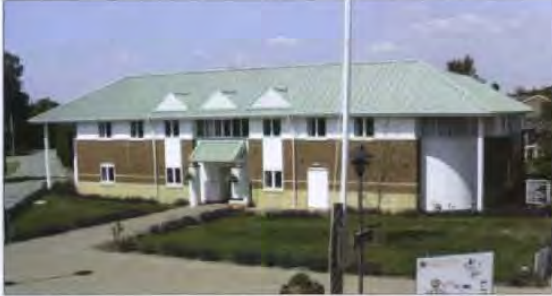
Alan Parton Building, Warwickshire College
