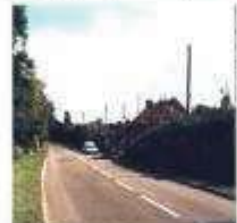
There is some unfortunate wirescape along the south side of Henley Road north end of Park Lane.
