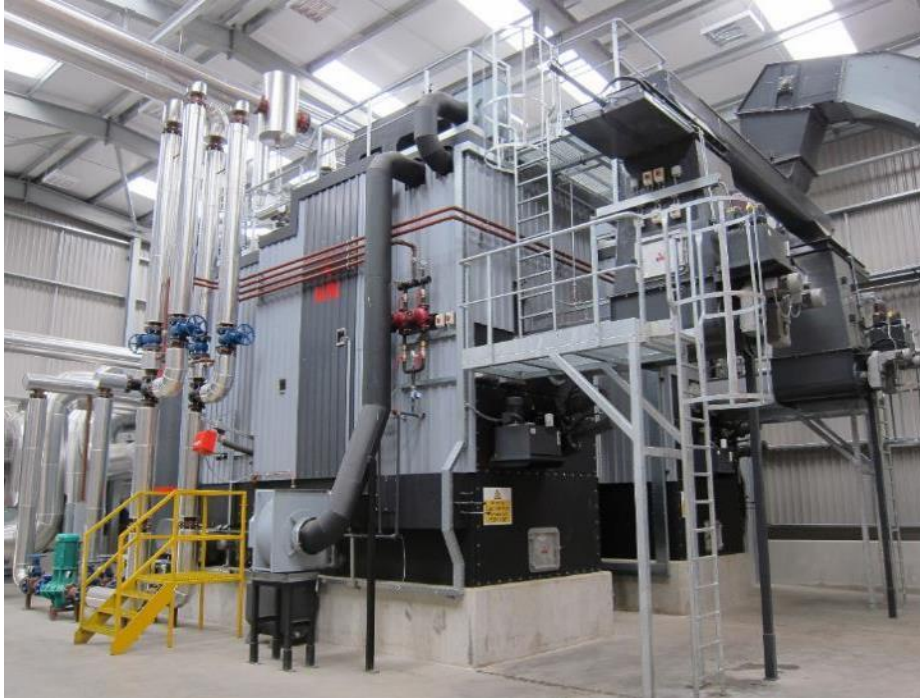
6MW Wood Chip Boiler at Sawmill Site in Mid-Wales, Photo Courtesy of Sustainable Energy Ltd
