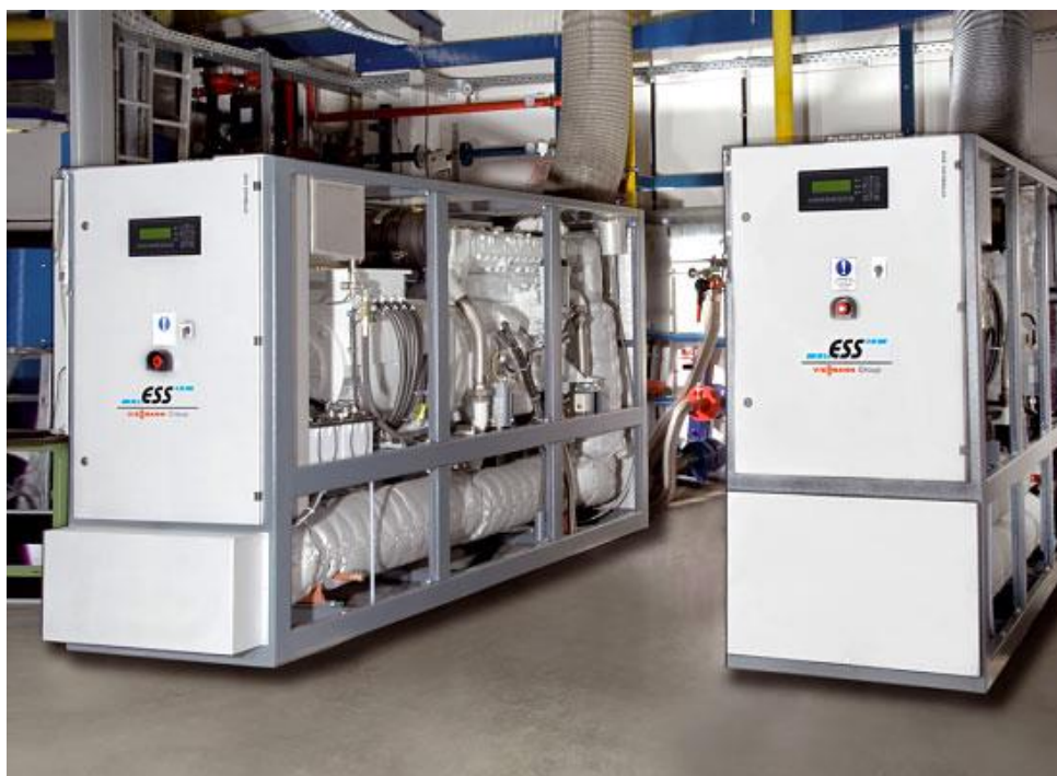
400kWe Natural Gas CHP Plant. Photo Courtesy of www.viessmann.co.uk
