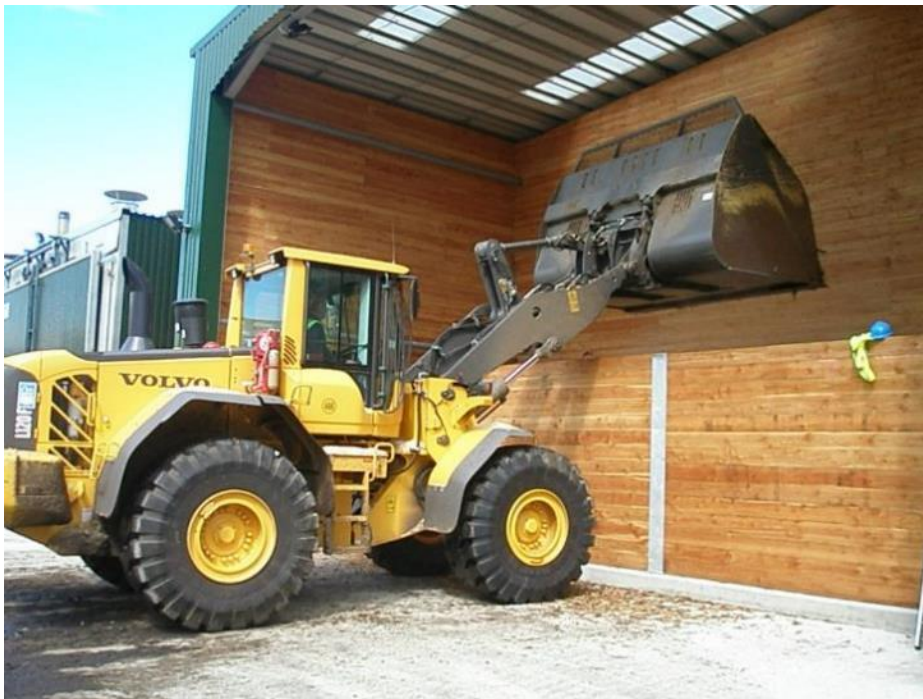
Wood Chip Delivery to Wood Chip Store for 6MW Biomass Boiler, Photo Courtesy of Sustainable Energy Ltd
