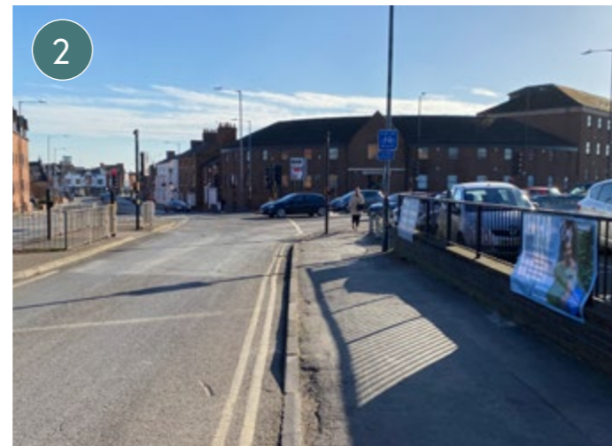
VIEW LOOKING TOWARDS THE SOUTH ALONG BIRMINGHAM ROAD
