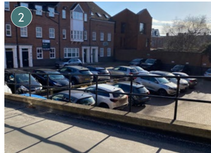
LOWER GROUND LEVEL PARKING
