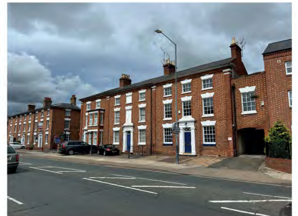
Figure 4.6 Georgian townhouses, Guild Street
