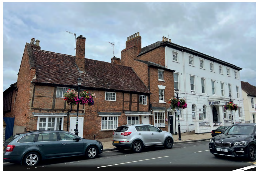
Figure 5.15 Civic Hall and 11, 12 and Rother Street
