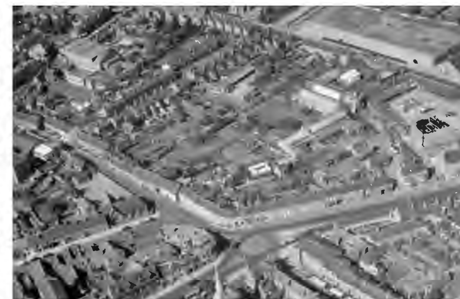
Figure 4.14 View of the Site from the north-east, 1951 (source: Historic England)
