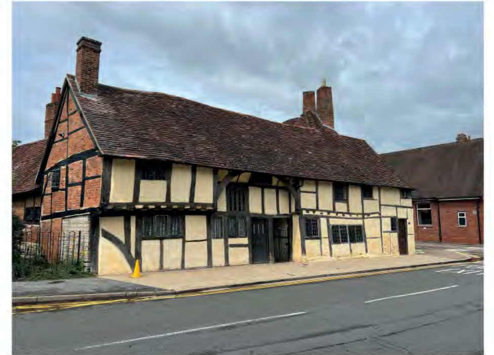
Figure 4.5 15th century timber framed Wealden House, Rother Street
